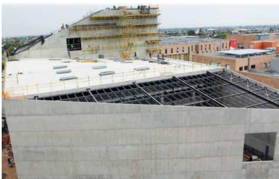
*This three-dimensional concrete envelope is functionally, structurally and technically separated from the inner core of the building*
